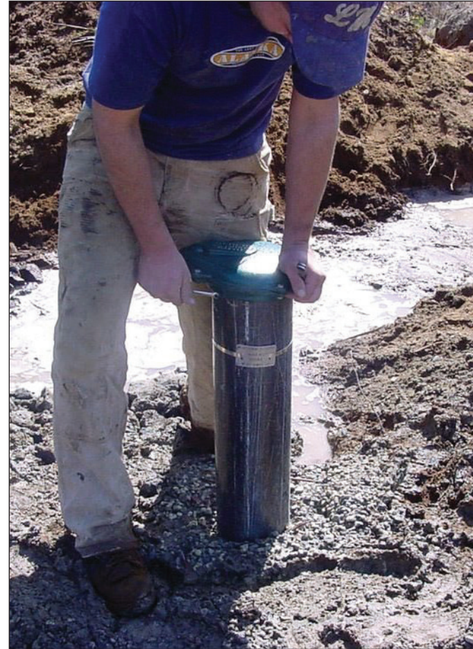
A well driller works on the end cap of a well. Photo courtesy of Department of Ecology
